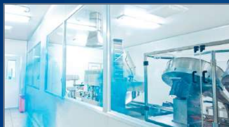
HVAC, Clean Room & Environmental Control Systems
